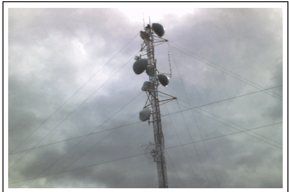
A Look at the Tower Holding the Mich-A-Con Repeater Antennas
